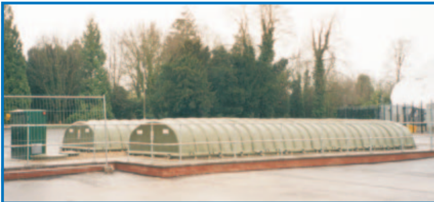
2 x F13 NuDisc® treating domestic wastewater for a Media Corporation
