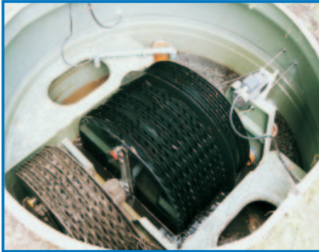
◀ NuDisc® showing Anoxic and Aerobic RBC stage.
